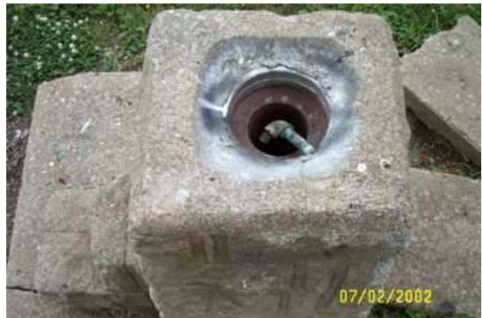
Fountain with missing faucet and no running water - Blenheim Park, 7/2/02
