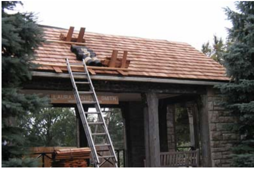
Made significant progress on restoring or replacing park structures
