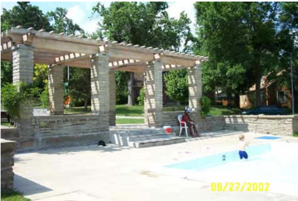
Structure with no problems - Arbor Villa, 6/27/02
