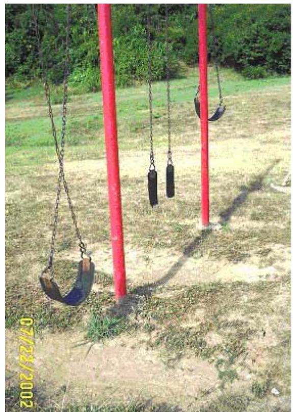
Twisted and broken swings with no soft surface underneath - Liberty Park, 7/22/02
