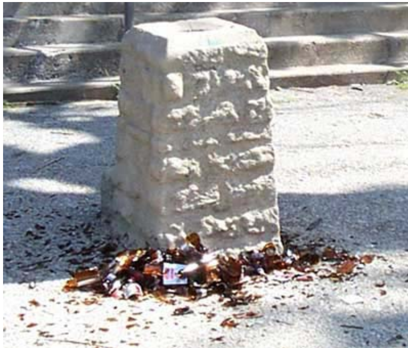
Broken beer bottles surround the base of drinking fountain - Budd Park, 7/1/02
