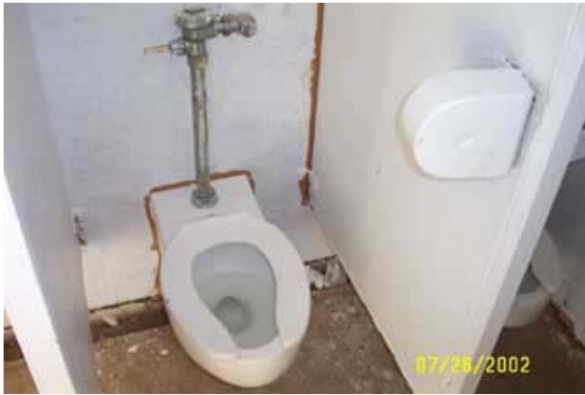
Clean toilet - Englewood Park, 7/26/02
