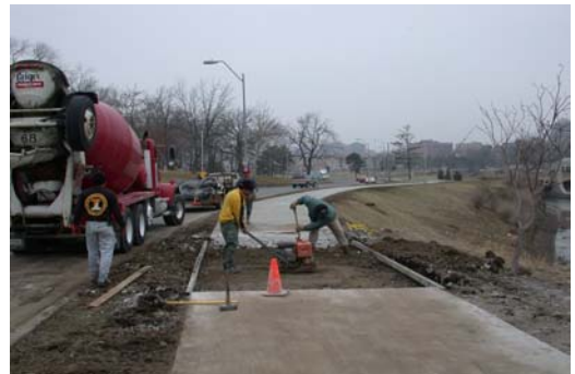
Replaced over 116,000 square feet of sidewalk and 12,000 feet of curb
