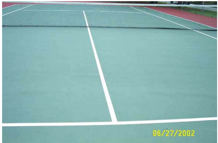
Tennis court surface with no problems - Arbor Villa, 6/27/02
