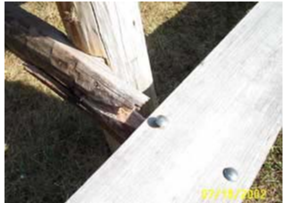
Picnic table with splintered crosspiece - Brookside Park, 7/18/02
