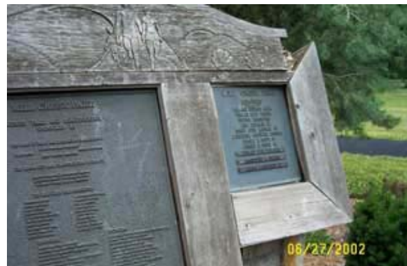
Rotted corner of the fitness trail dedication sign - Mill Creek Park, 6/27/02
