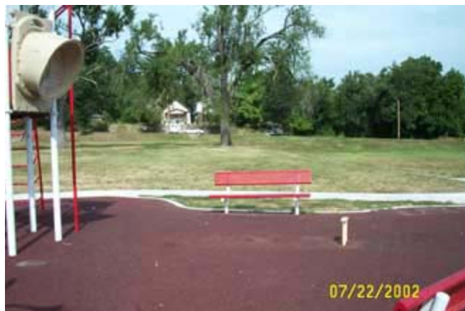
Tube slide missing from playground - Ashland Square, 7/22/02
