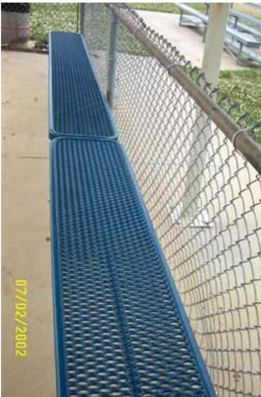
Dugout bench with no problems - Cleveland Park, 7/2/02
