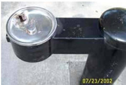
Damaged and inoperable drinking fountain - Lykins Square, 7/23/02
