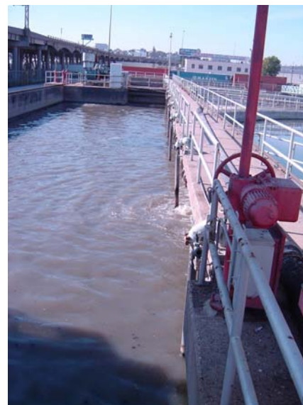
Aerated Grit Removal – Westside WWTP
