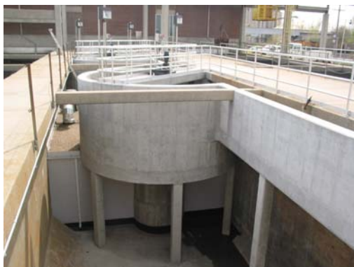
Vortex Grit Removal - Blue River WWTP
