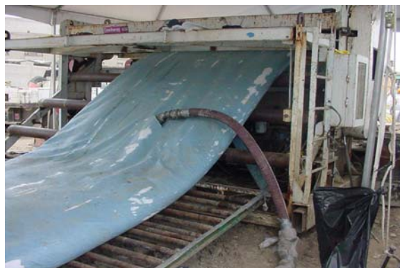
Freight-House – Cured in Place Pipe
