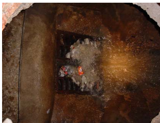
Flow Regulating Structure - Grating
