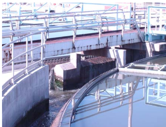
Primary Clarifier Weir – Westside WWTP
