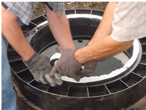
Applying Manhole Riser Sealant
