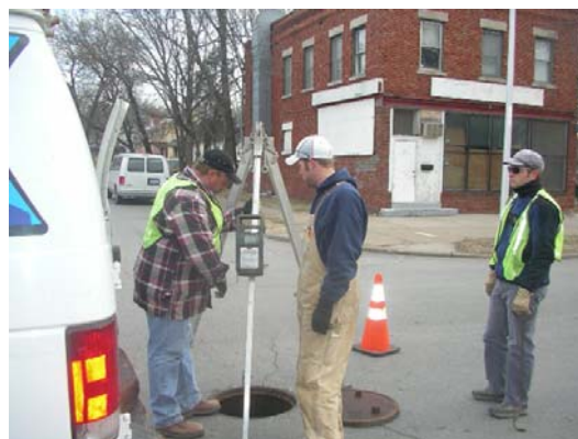
Temporary Flow Metering – Confined Space Entry
