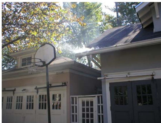
Smoke Testing to Check Roof Drain Connection
